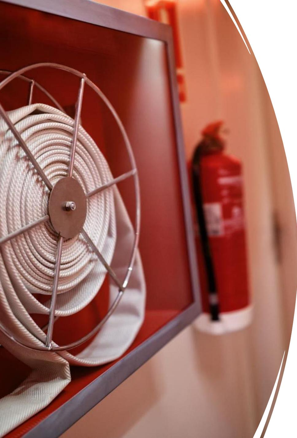
A circular inset image on the left side of the slide. It shows a fire hose reel with a white hose coiled on a metal frame. In the background, a red fire extinguisher is visible on a wall.
