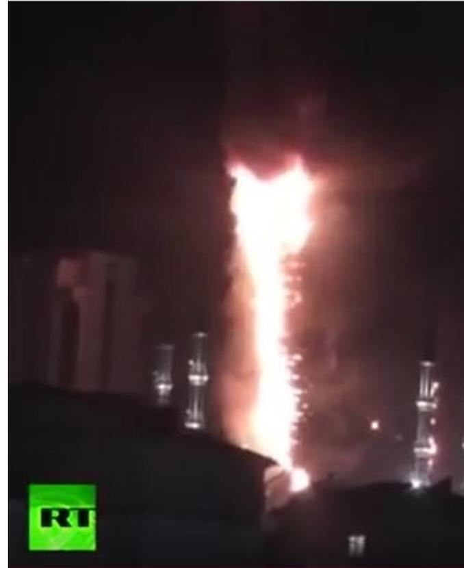
Downward fire spread with an inclined (diagonal) front
