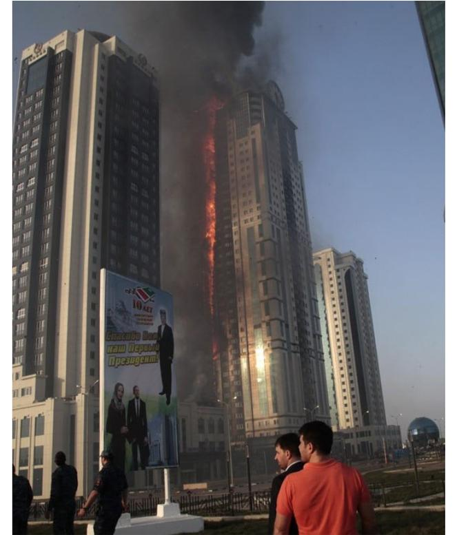
Upward fire spread with an inclined front
