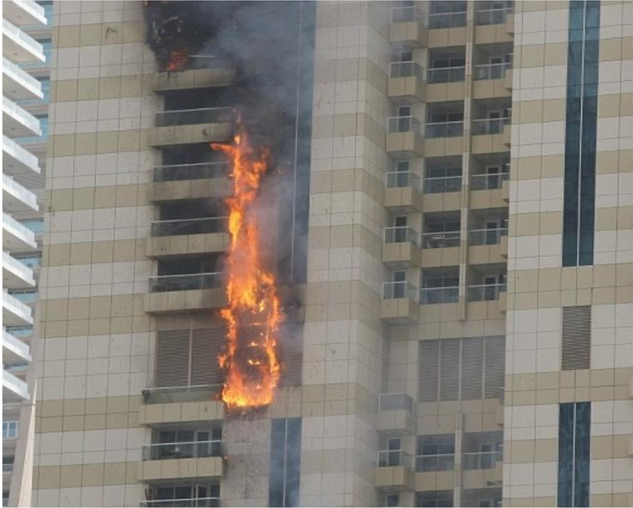
Upward vertical fire spread
