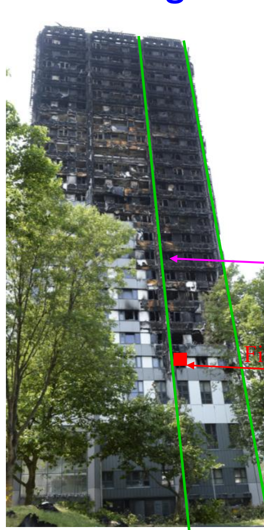
the Grenfell Tower
