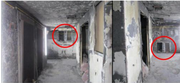
Lobby vents in GT (were not active during the GT fire, Lane, 2018)
