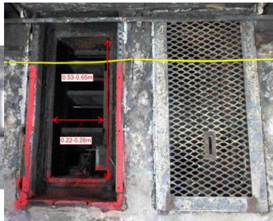
Lobby vents in GT (were not active during the GT fire, Lane, 2018)
