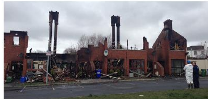
Figure 2. Fire stopping / compartmentation omitted.
